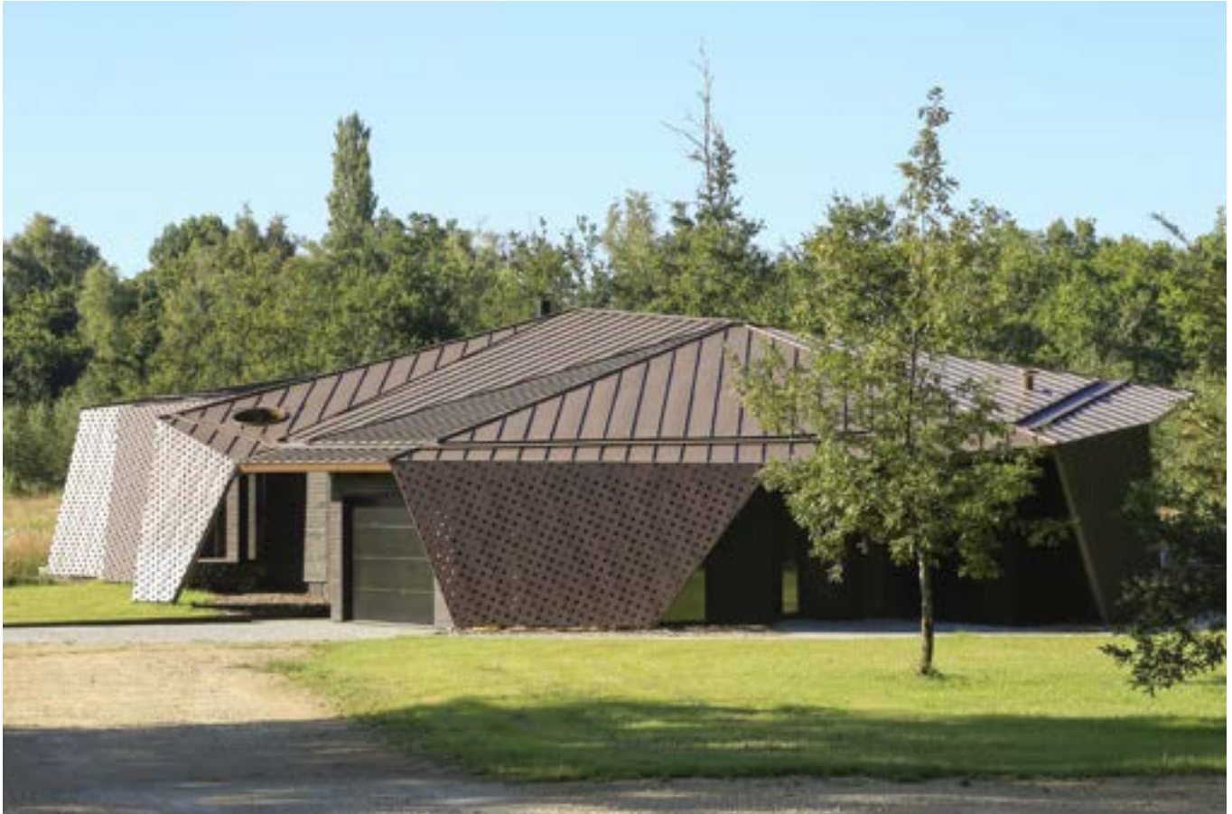
Single-family home, Mezos (France) - Architect: Latour Salier - Bordeaux 33 - Technique: VMZINC® Standing seam.
