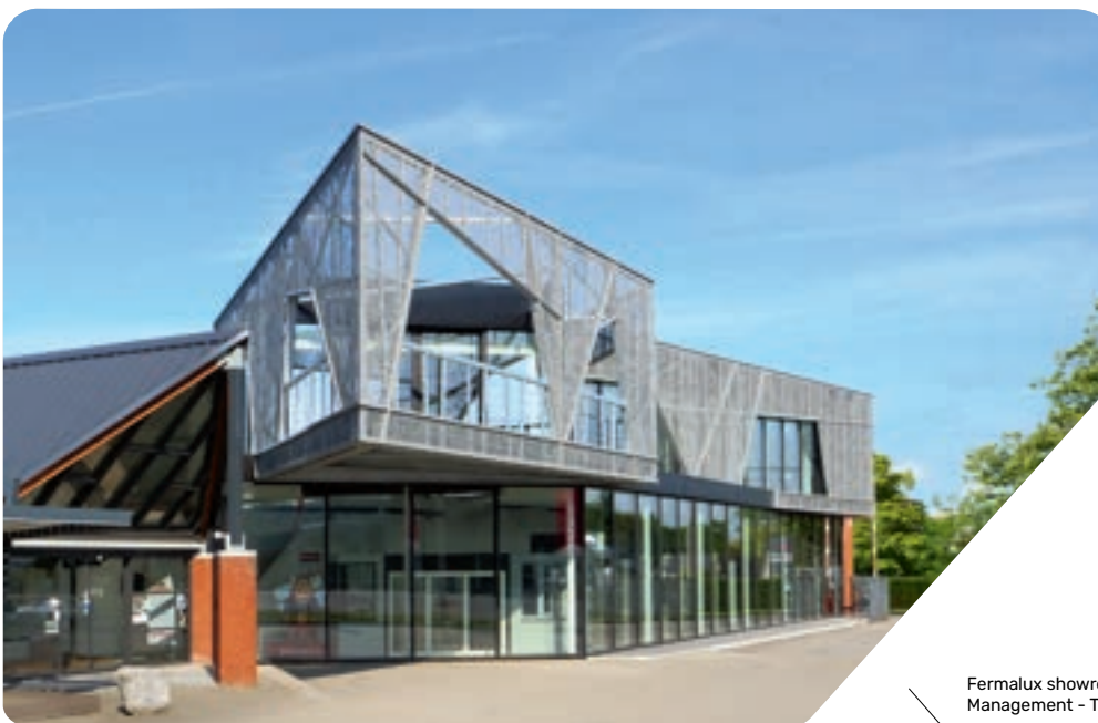
Service centre, Castelnau Pegayrols (France) - Architect: Christophe Cartayrade - Technique: VMZINC® Standing seam and VMZINC® Interlocking panel.
