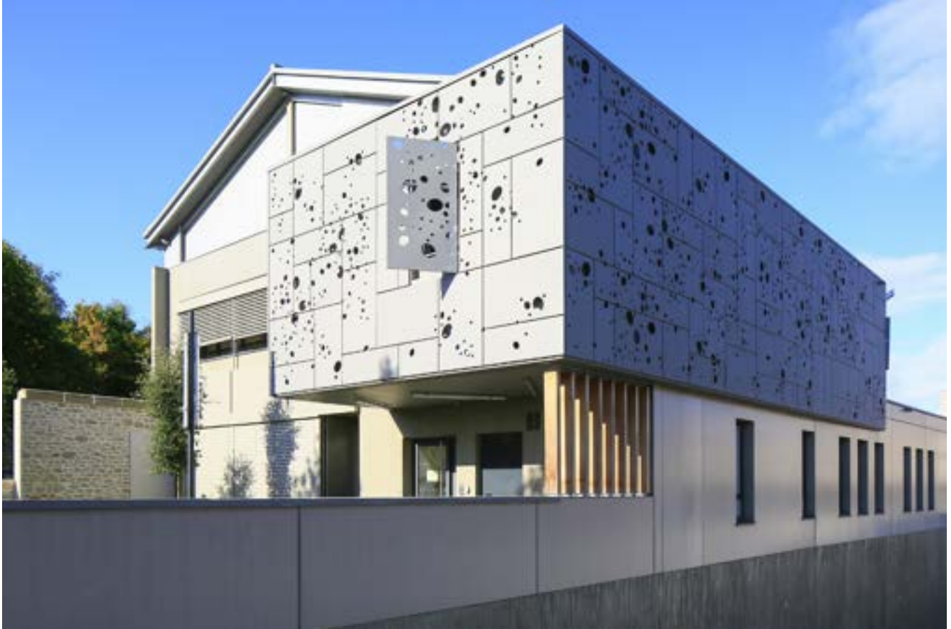
CPAM, Dinan (France)- Architect: Ateliers cub 3, Liffre 35 - Technique: VMZINC® Standing seam and MOZAIK®.
