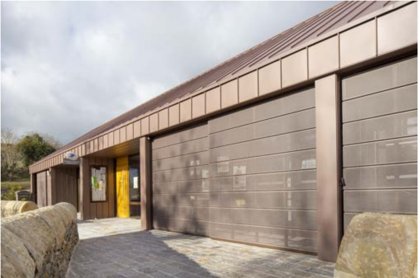
Service centre, Castelnau Pegayrols (France) - Architect: Christophe Cartayrade - Technique: VMZINC® Standing seam and VMZINC® Interlocking panel.
