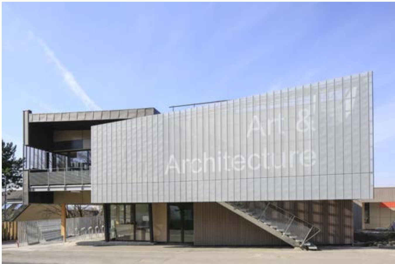
Gustave Eiffel high school, Gagny (France) - Architect: Marc Nicolas Architectures - Montrouge 92 - Technique: VMZINC® Interlocking panel.
